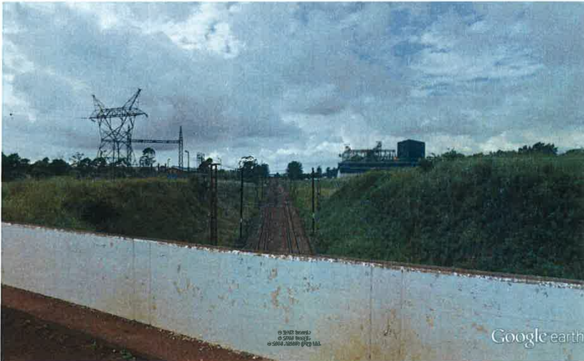
Fig. 8 –View of railway crossing site proposed by alternate route 2 (point 5)
