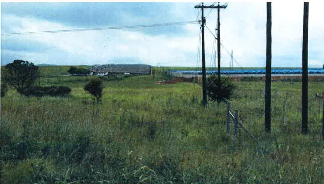
Fig. 11 – Car ports constructed on Erf 885 Portion 114 Vaalkop & Dadelfontein
